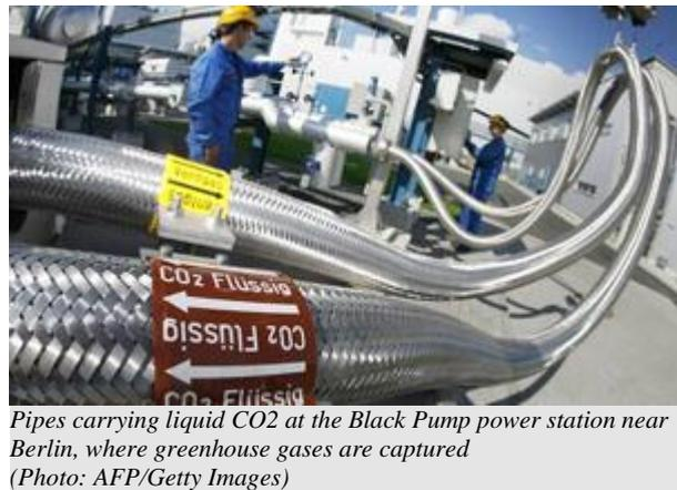
Pipes carrying liquid CO<sub>2</sub> at the Black Pump power station near Berlin, where greenhouse gases are captured
